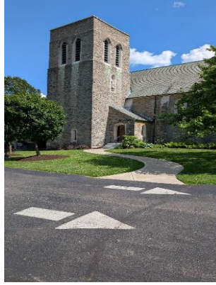
Carillon Tower Convent of the Transfiguration
